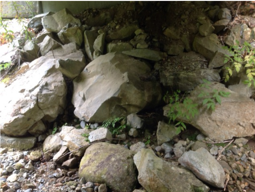
Right Bank Abutment when facing downstream
