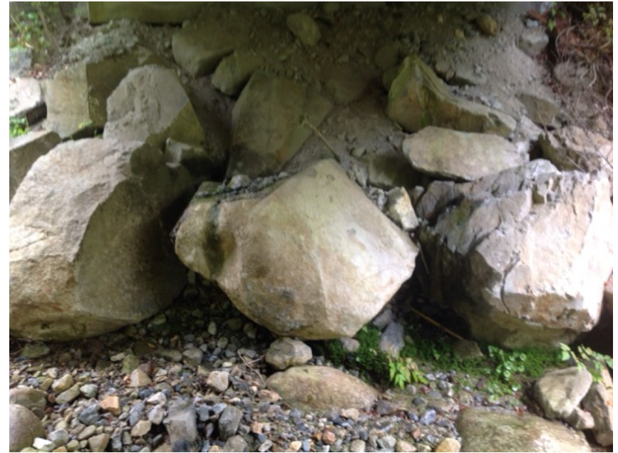
Left Bank Abutment when facing downstream
